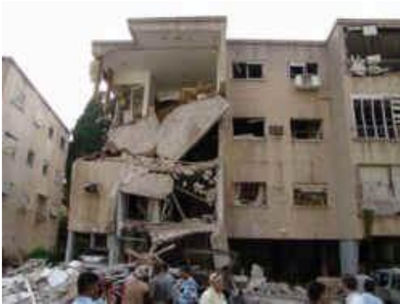
Building destroyed in Israel vs. Hezbollah 2006 Haifa, Lebanon 2007
